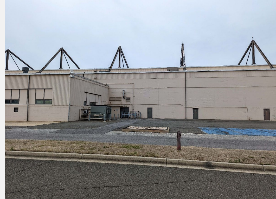
Site of new concrete loading dock
